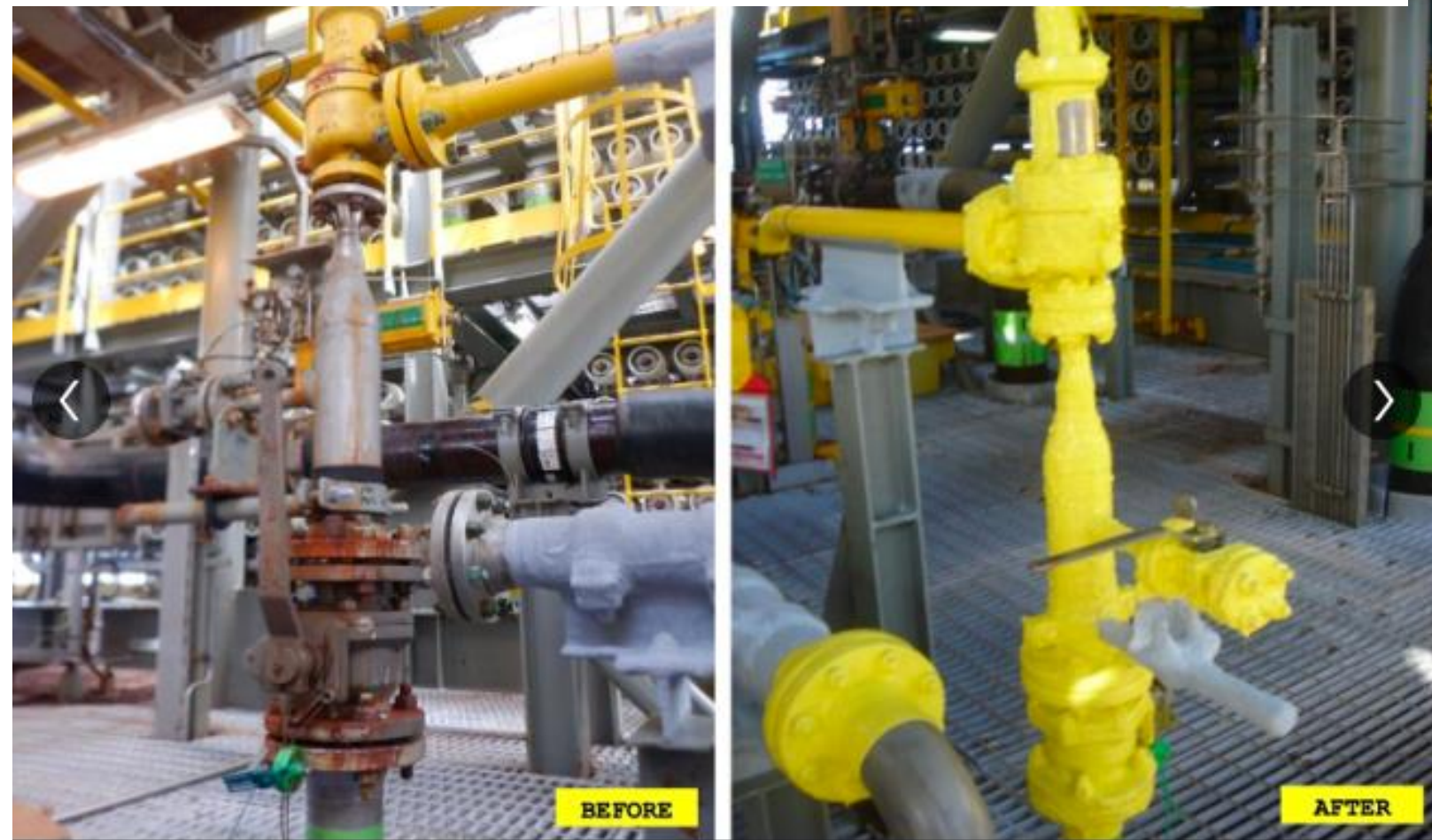
FLANGE: Protecting flanges and stud bolts/nuts from corrosion.
