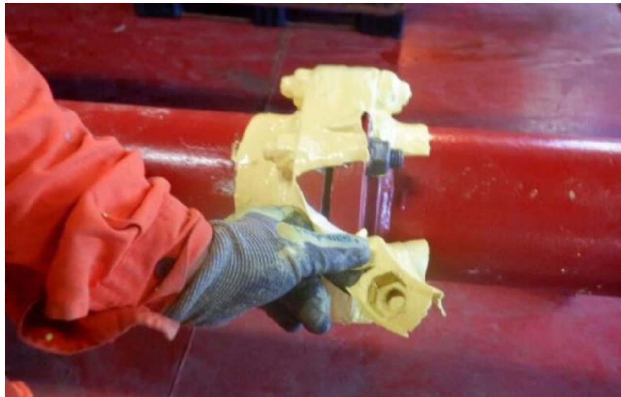
FLANGE: Protecting flanges and stud bolts/nuts from corrosion.
